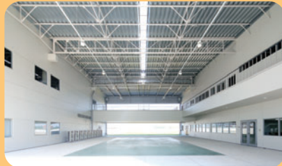
Sports area inside the plant grounds
