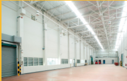
Plant using natural lighting
