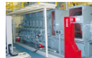
Kagoshima-Miyanojo Factory co-generation power generator
