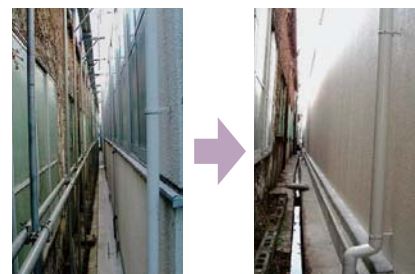
Sound barrier installed at Nittoku Seisakusho
