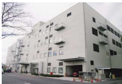
No. 1 Plant Building of Komaki Factory
