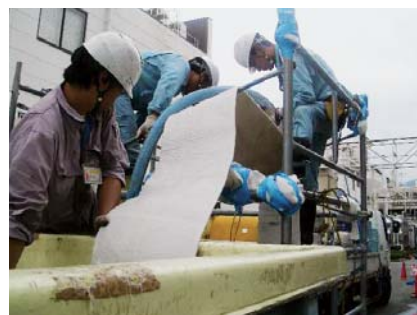
Sewage pipe reinforcement work
