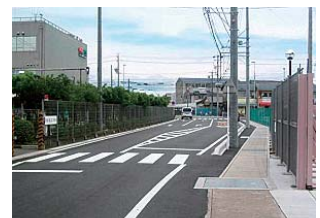
The new right-hand turn lane
