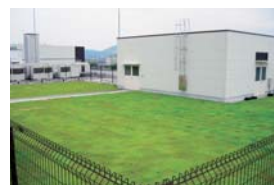
Rooftop greening (Komaki Factory)
