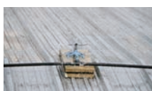
Energy Saving Measures
